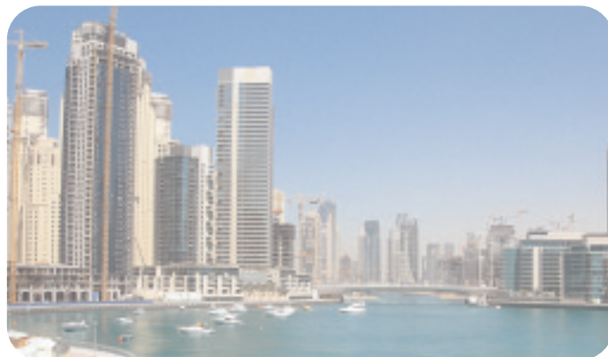
The Dubai Marina currently under construction
